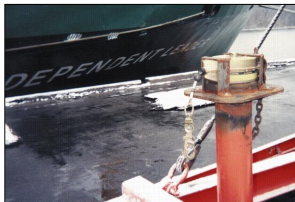
Figure 92 End pillar anchorage for personnel protection.
