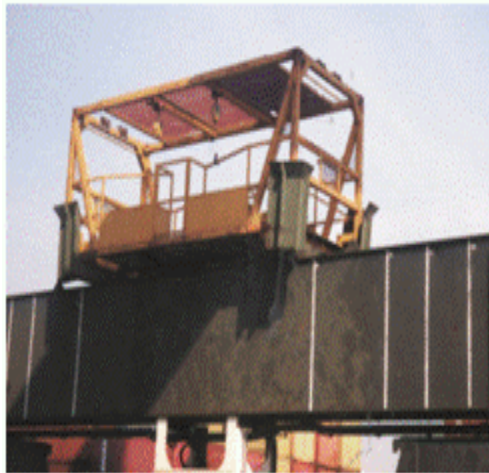
Figure 66 20 ft personnel cage stowed on cill of container crane.
