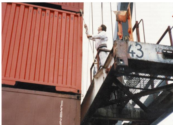
Figure 54 Work from a platform on a spreader.
