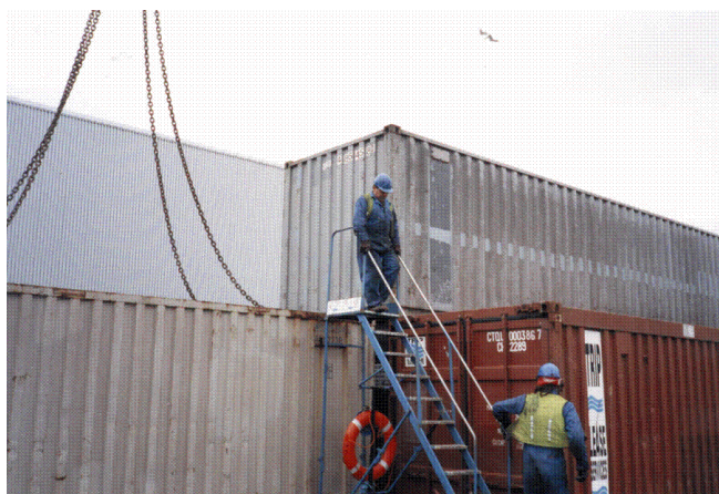
Figure 53 Mobile step accesses to containers.
