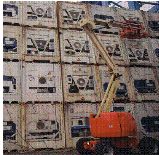
Figure 49 Use of MEWP to access Containers.
