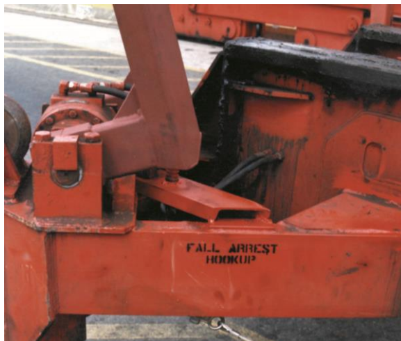
Figure 110 Identification of fall arrest anchorage location on spreader.
