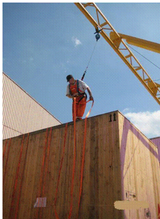
Figure 90 Worker on top of case protected from mobile frame.
