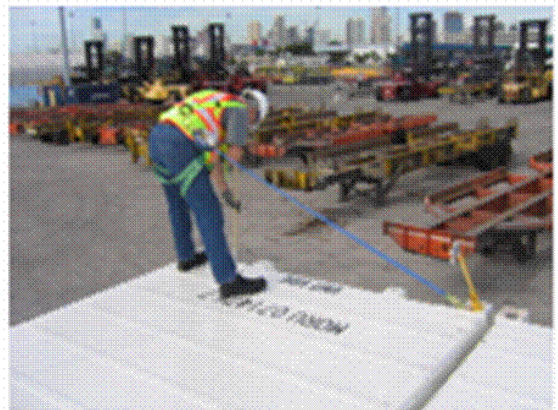
Figure 87 Working attached to Top Lock Container Wand.
