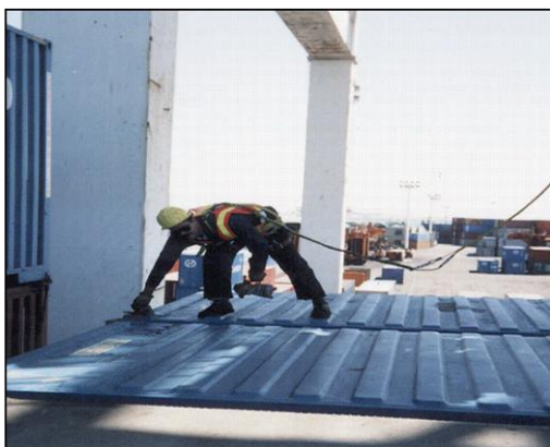
Figure 76 Work on top of containers while protected. Note 'fuse' to limit forces on man and harness in the event of a fall
