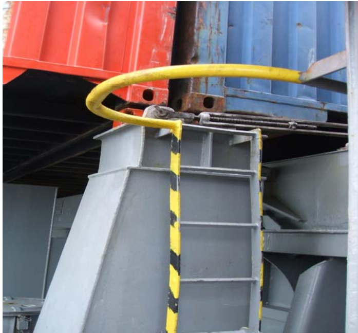
Figure 9: Lack of working platform
