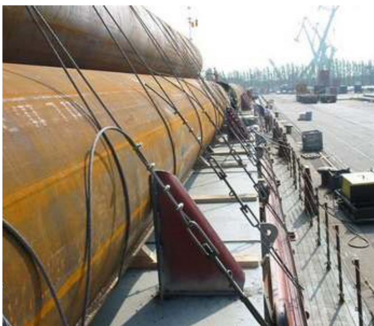
PICTURE 1 Wire lashings used to secure pipes on deck
