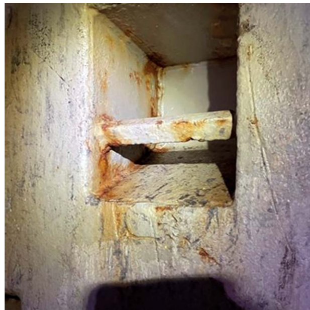
Figure 1: A recessed foothold
