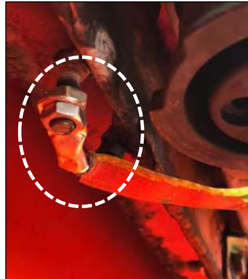
Figure 4: Earthing connection after renewal
