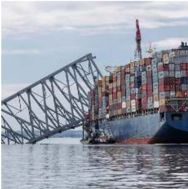
Study: bridges may need more protection from ship collisions
