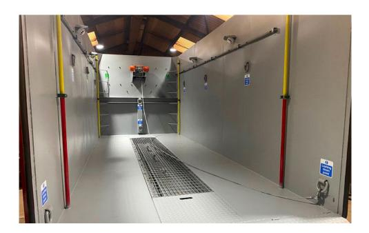
The EVCU, specifically designed for vehicles, provides a secure environment to transport, and store electric vehicles, minimising fire risks and providing immediate deployment of firefighting capabilities on detection of a fire.
