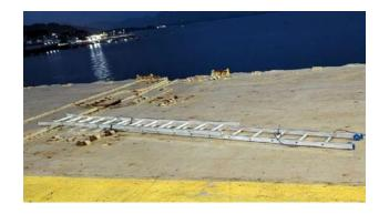
Incident 3: This ladder was used to access the top of plywood cargo on deck. Nobody was holding it. The ladder slid and the person using it fell from a height of about 2 meters.
