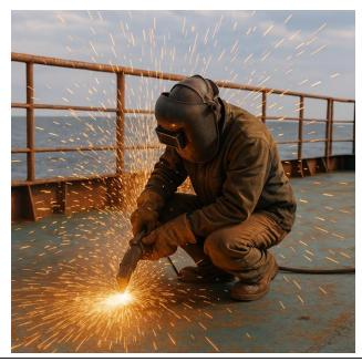
If the deck is penetrated by accident, or overheated, a fire can start in the space below.
