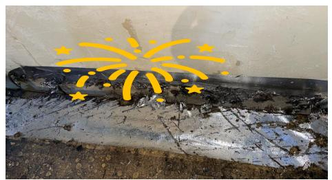
1. Flame retardant tape was used to cover the gap between bulkhead and tween deck. Sparks from hot work melted through the tape.
