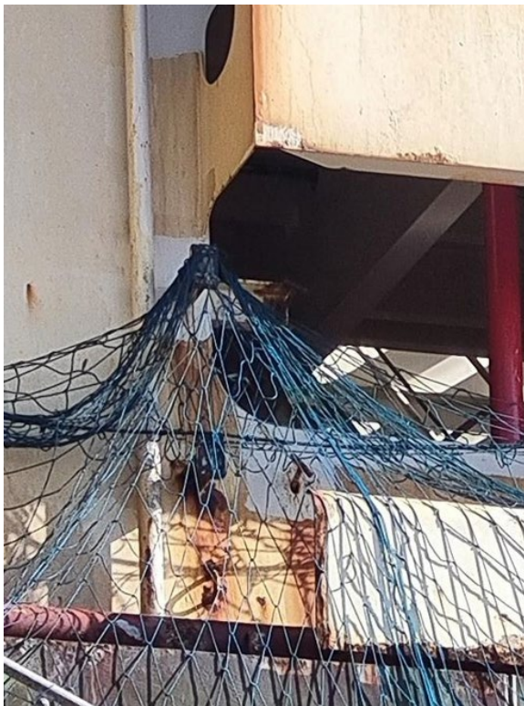
Net hanging from a bracket. Not tied off and potentially damages the net
